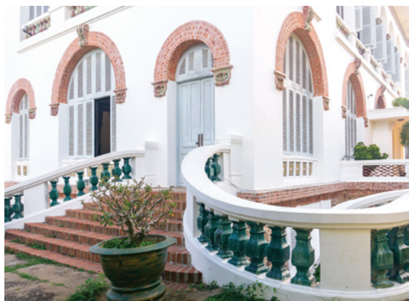
The staircase features green ceramic balustrades
